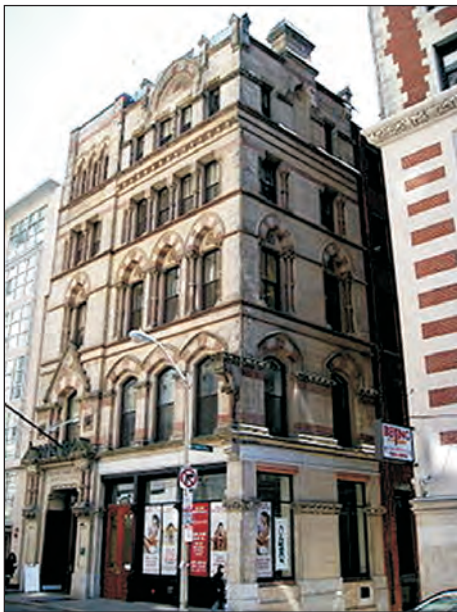
Sammy Lyman and his wife, Kate, lived for many years in an apartment at the Young Men's Christian Union at 48 Boylston Street in the heart of Boston's rundown theatre district. Today the 1876 building is on the National Register of Historic Places, and houses the Boylston Street Athletic Club. In the late 1940s its gym was known as the practice and meeting space for Boston-area amateur and professional jugglers.
